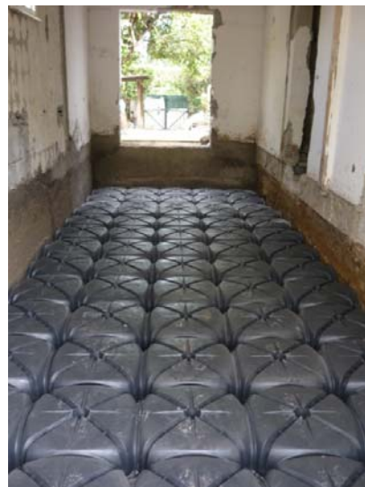
Renovation of an existing house outside of Rome using ventilated under-floor cavities. This feature enhances energy efficiency, reduces dampness, mold and mildew, and diverts any permeating gases (including radon) to the outside of the building. The theory behind this new system is based on the structural characteristics of the ancient dome
