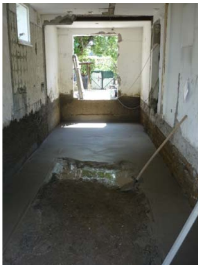
Renovation of an existing house outside of Rome using ventilated under-floor cavities. This feature enhances energy efficiency, reduces dampness, mold and mildew, and diverts any permeating gases (including radon) to the outside of the building. The theory behind this new system is based on the structural characteristics of the ancient dome
